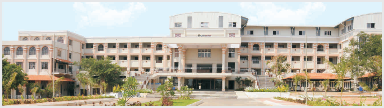
PMC TECH - Engineering Main Block
